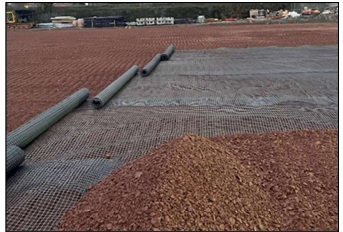
Figure 6: Placement of granular backfill and geogrids
