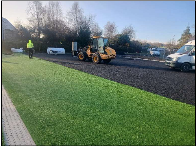
Figure 10: Installation of blinding, shock pad and carpet
